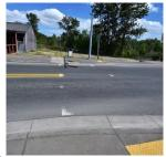
Benton County Public Works Staff has starting applying Thermoplastics striping to the 16 existing crosswalks along Hwy 99 within the city limits. Thermoplastics is more than just painting the crosswalk lines as this process involves a matting process which will make the results last longer (about 5-7years) and not require an annual re-paint.
