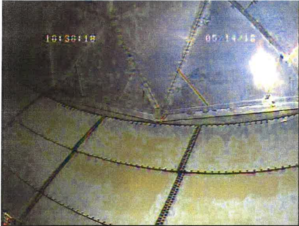
Wall to Roof Seam
