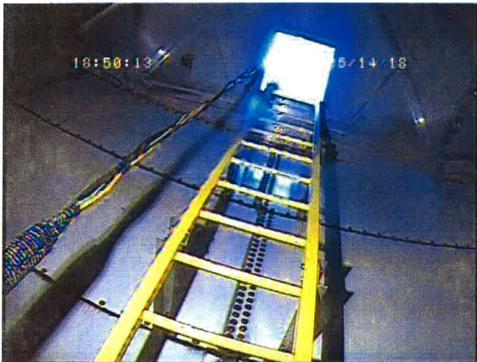
Interior Ladder and Access Hatch
