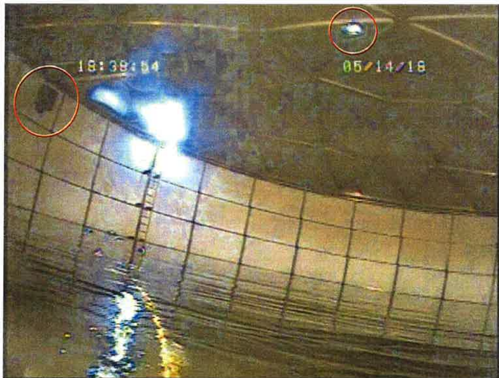
Typical Roof, Vent, and Overflow
