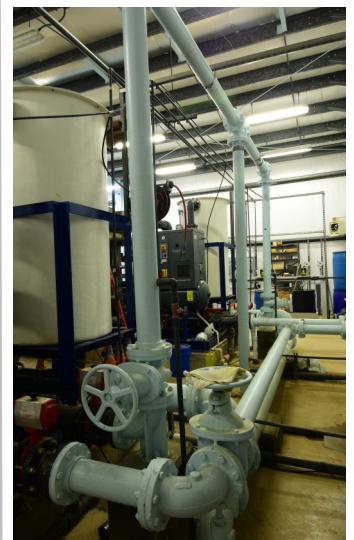
Inside the water treatment plant
